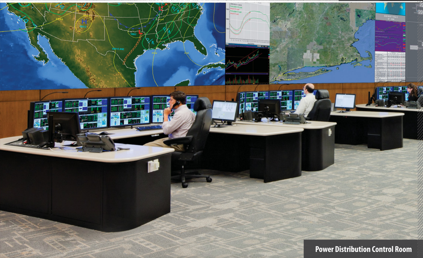
Refinery Control Room
