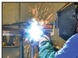
Frames are welded together
