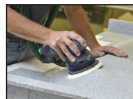
Final buffing and finishing onsite during installation
